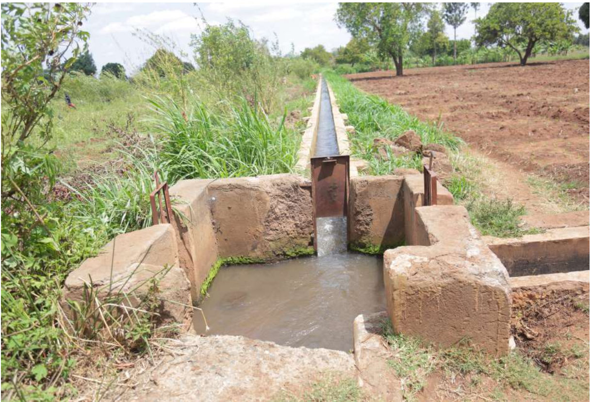
Lined canals with spring water for irrigation in Njukini Irrigation Project
