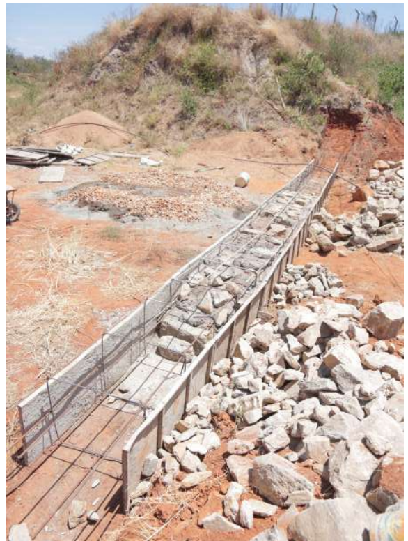
Construction of a sill at Kyamusoi Community water pan in Makueni County
